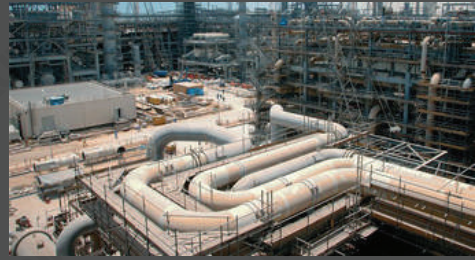
DUBAI : BARZAN ONSHORE FACILITIES PROJECT IN RAS LAFFAN, QATAR
