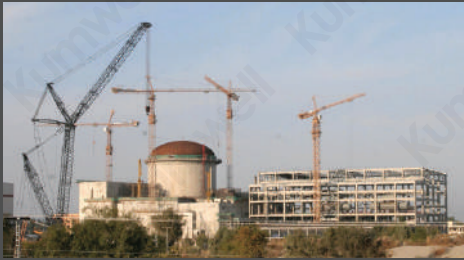
CHINA : 6100 MW YANGJIAN NUCLEAR POWER PLANT
