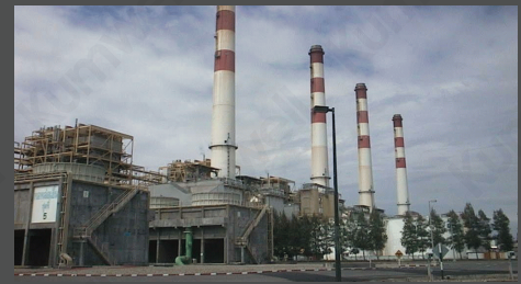
THAILAND : PTT GASSEPARATION PLANT
